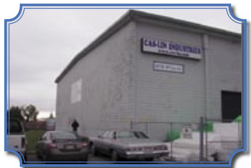
Building exteriors - To remove peeling paint in preparation for painting
